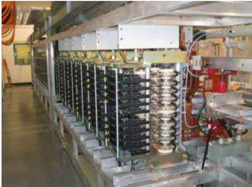
BESS installation in Fairbanks, Alaska
