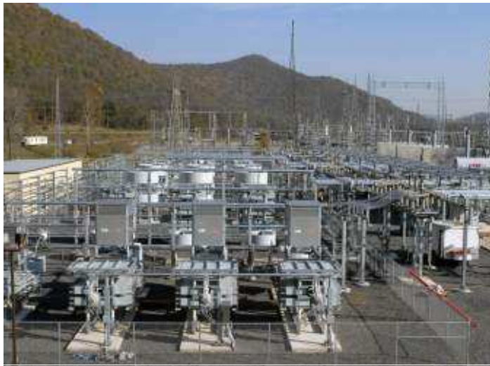
The world's largest SVC with 500kV, -145 /+575 MVar at Allegheny Power/US delivered by ABB
